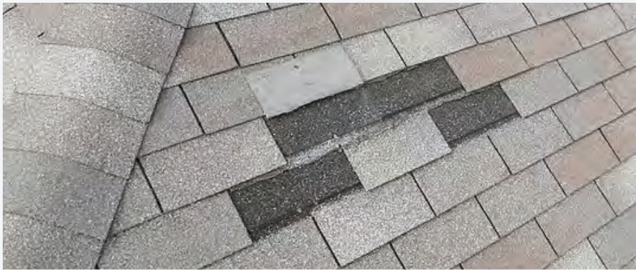
MISSING SHINGLES
